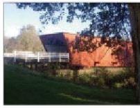
ROSEMAN (over Middle River) BRIDGE 1883
