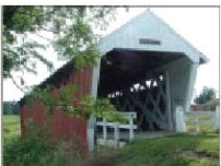
IMES COVERED BRIDGE 1870
